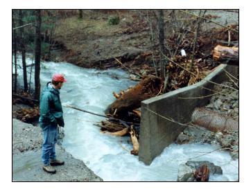
Figure 5-7. Culverts Will Inevitably Plug With Debris. Critical Dips At Crossings Will Ensure That Flows Remain In Stream Channels.
