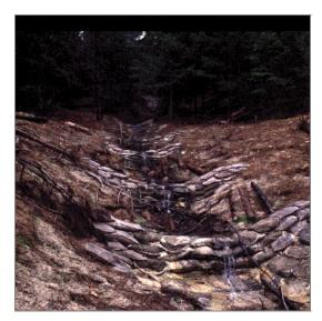
Figure 5-10. Soil/Cement Checkdam
