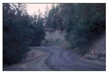
Figure 5-5. Outsloping Reduces Concentrated Flow on Road Surface
