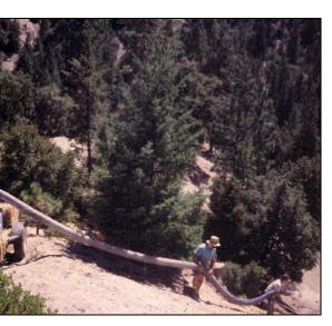
Figure 6-18. Using Straw Blower to Apply Mulch
