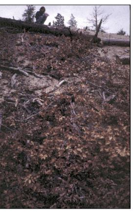
Figure 6-9. Slash Spread on a Sheet and Rill Slope
