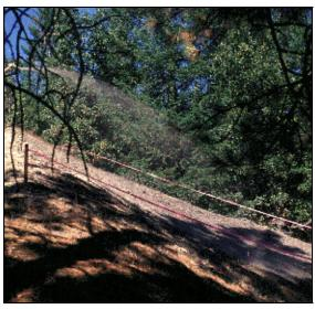
Figure 6-17. Lime-Based Tackifier Being Applied
