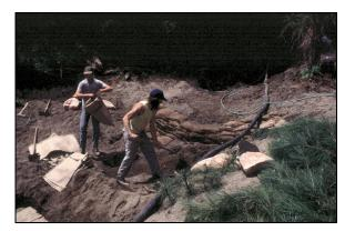
Figure 3-6. Grade Stabilization Structures are Incorporated into most Road-Crossing Excavations
