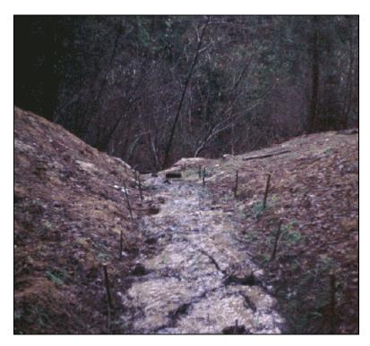
Figure 6-7. Willow Stakes Installed Along an Excavated Channel
