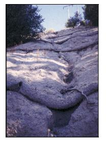
Figure 6-13. Straw Wattle on ORV-Damaged Site
