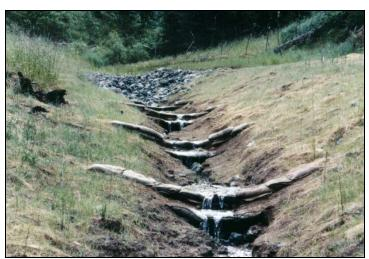
Figure 3-2. Soil/Cement Grade Stabilization Structure.
