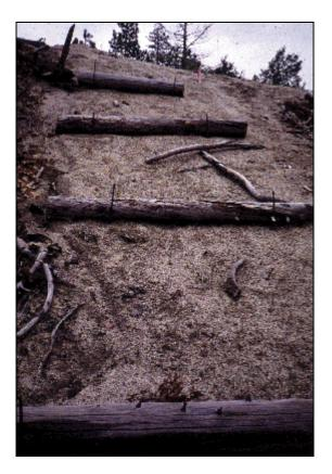
Figure 6-15. Cross Slope with Logs
