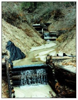
Figure 3-1. Log Grade-Stabilization Structure
