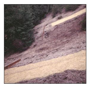
Figure 6-16. Erosion Blankets
