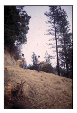
Figure 6-2. RCD Crew Spreading Mulch
