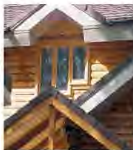
Enclose eaves and soffits.
