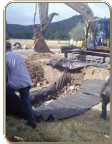
Four rock "checks" were constructed upstream of inlet to ease gradient.
