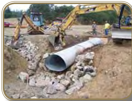
Placing of the new culvert
