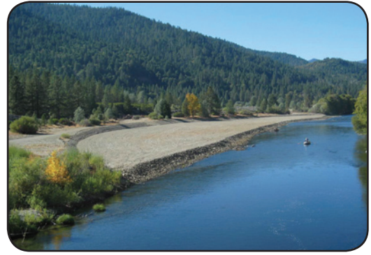
Hocker Flat, Post Construction at 450 cfs Flow.
