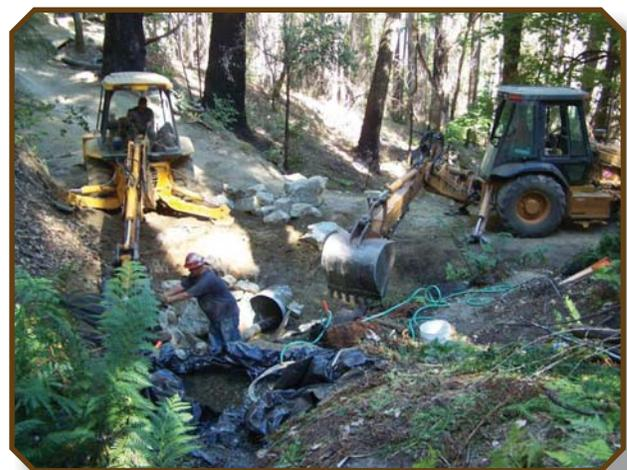
**Temporary stream diversion for culvert installation**
