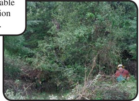
Clearing out low branches and brush along roadway reduced risk for flames to spread, helping make this area fire safe. TCRCD crews chipped much of the cut material.
